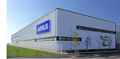
An expanded hangar building at Kobe Airport
