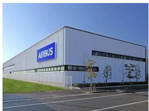
An expanded hangar building at Kobe Airport
