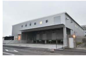
A warehouse at the Technical Center
