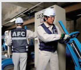
給排水施設のメンテナンス Maintenance of water supply and drainage facilities
