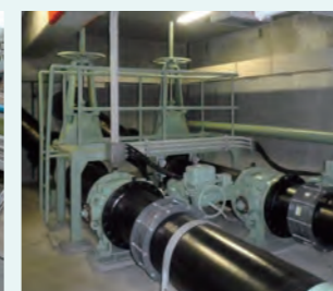
給排水施設 Water Supply and Drainage Facilities
