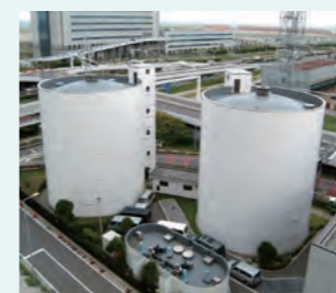
給排水施設 Water Supply and Drainage Facilities
