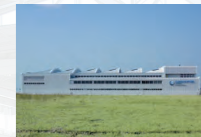
自然採光の窓と太陽光パネルを多数設置 There are many windows to take in daylight and solar panels installed.
