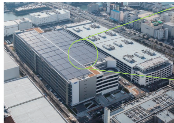
TRC Distribution B Bldg. rooftop solar power plant
