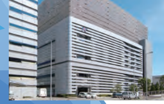
36 Addition to Maintenance Center No. 3
