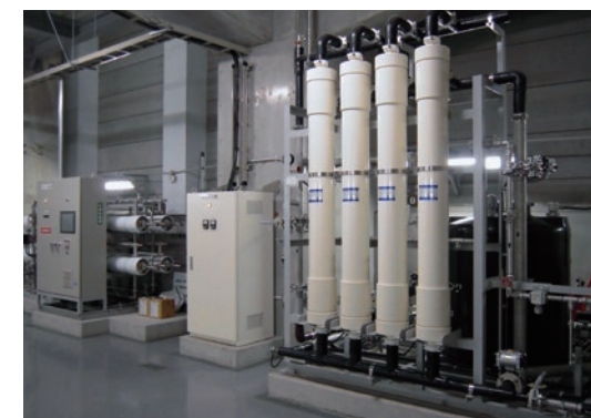
Water-saving cooling water recycling equipment
