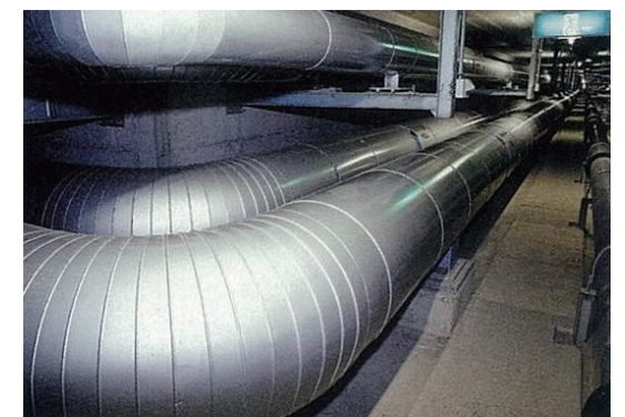
Pipeline (in public conduit)
