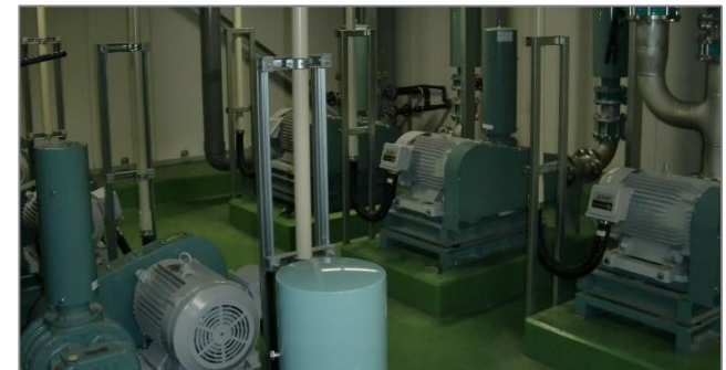
Inside view of the facility
