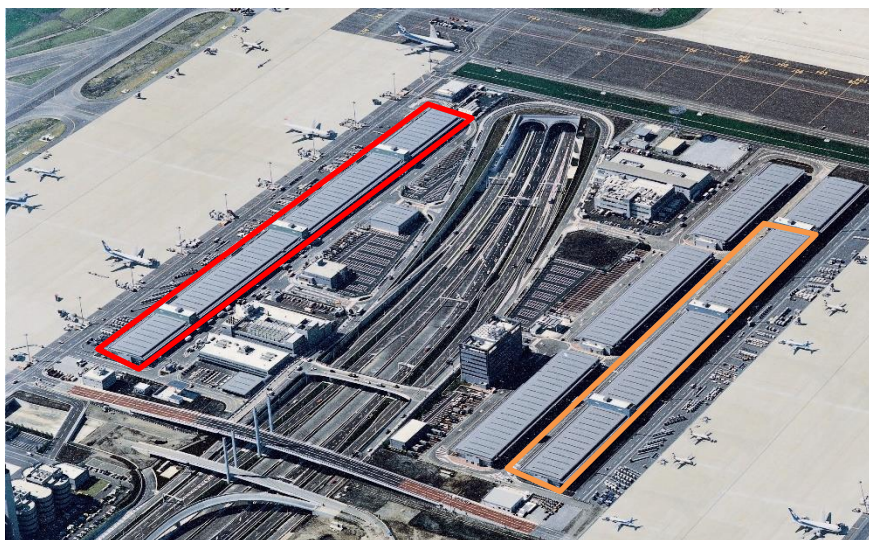
[Aerial photo of the Cargo Terminal Area of Haneda Airport] (Inside red line: W-1 Building; Inside orange line: E-4 Building)
